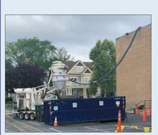
The large specialized truck in the photo is a Hydroexcavator used to remove the 10,000 square feet of gravel that covered the old roof.
