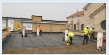
Ward roofers installed the new roofing material while torching the seams together.
