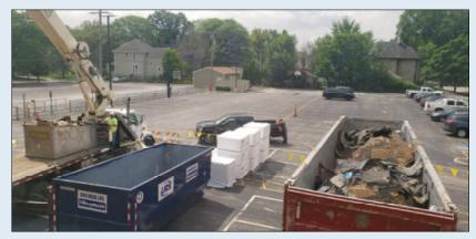
The dumpster contains the old roof materials, and sheets of insulation await being lifted to the rooftop.
