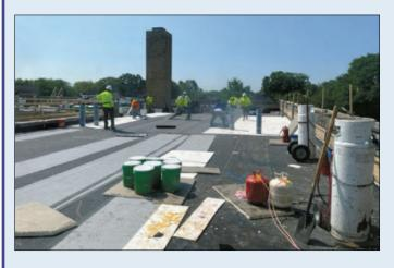
The crew layers the insulation onto the roof in order to pitch it correctly for proper drainage.
