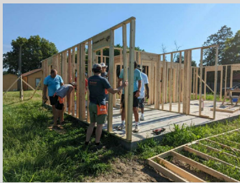
working on the walls
