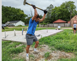
It started with a sledgehammer and a slab
